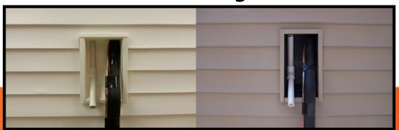
HVAC contractors now you have a termination point for your line set condensation drain & low voltage wire.
